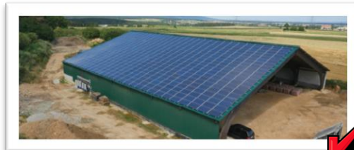
300 KWp in Ternitz
